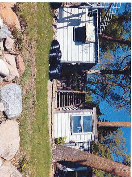
Sheds 9 & 10. View looking W.
